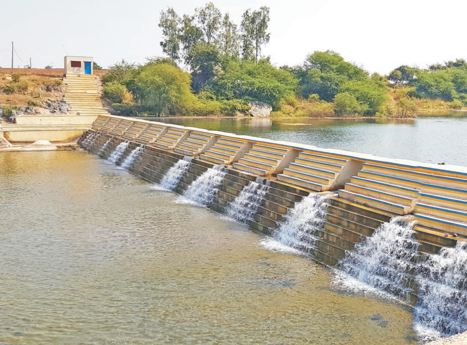
Bhatmahudi check dam across river Hiren Constructed under RKVY in Kushalgarh tehsil of Banswara district. Total storage of this check dam is 16 mcft, providing access to irrigation in 300 acres of land
