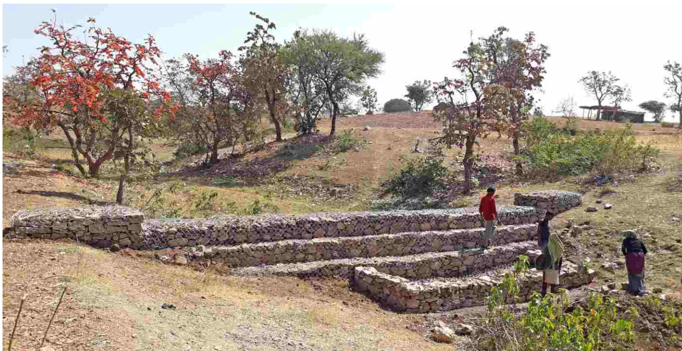
Gabion structure constructed in Kudla village under IWMP-10 Programme in Jhabua District.
