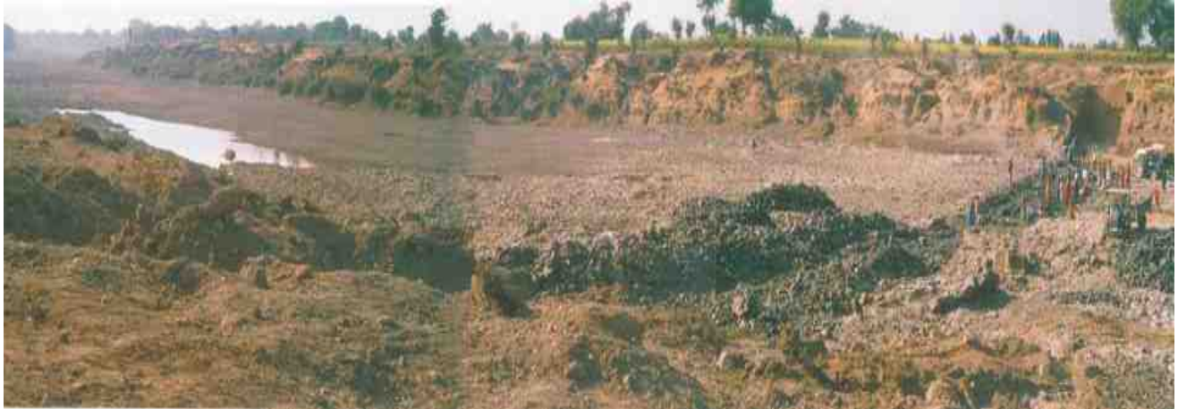
Initial stage of work - January 2005
