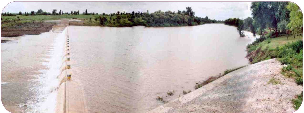
Karawan Check Dam on river Ahu under SGSY special project-II phase, Jhalawar, Rajasthan, designed and executed by N M Sadguru Water and Development Foundation.
