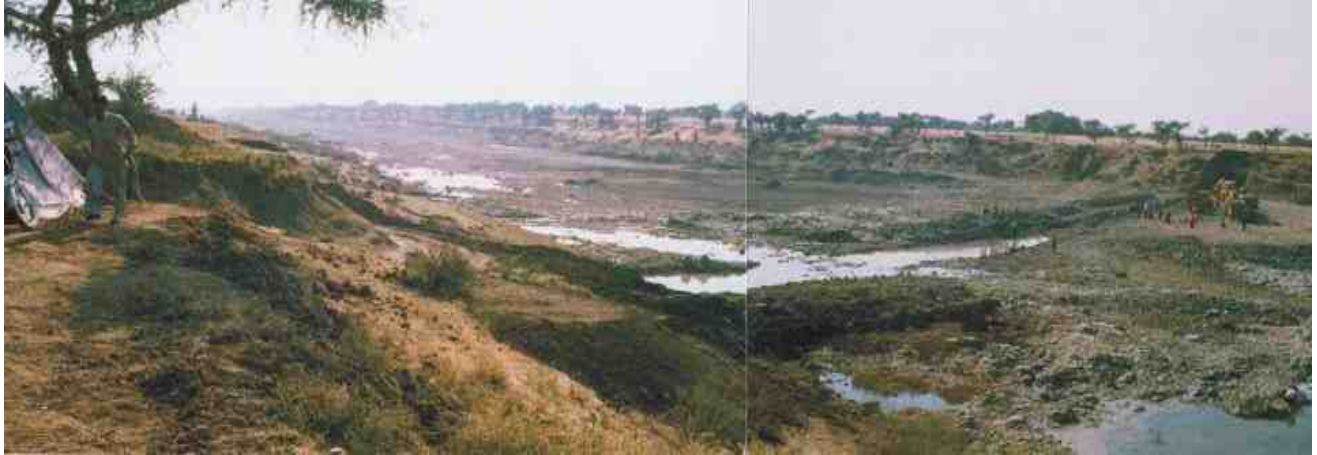
Initial stage of work - January 2005
