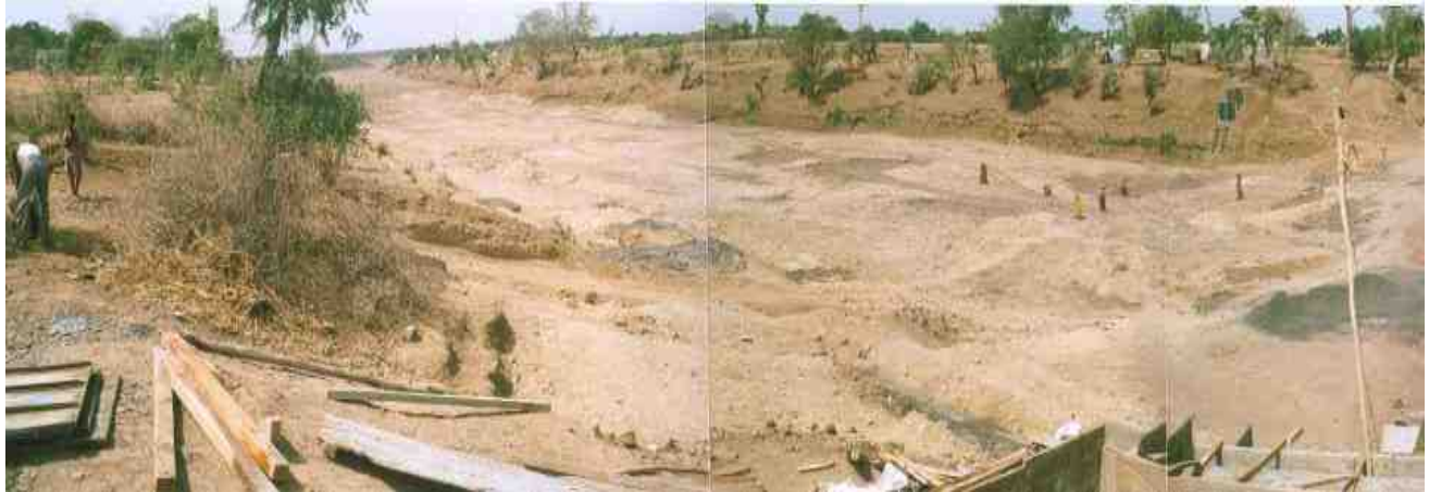
Initial stage of work - January 2005
